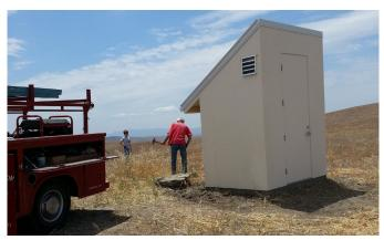
Figure 2.34.3. Installation of the surface hut at TRAM. Solar panels will be mounted on the south-facing roof. The door is 8 ft tall to allow access for installation of borehole equipment.
